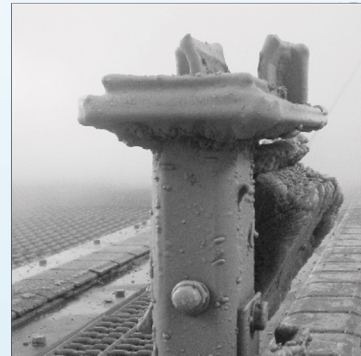
PAINT BOOTH & SKID CLEANING
