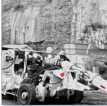
COAL FACE DRILLING
