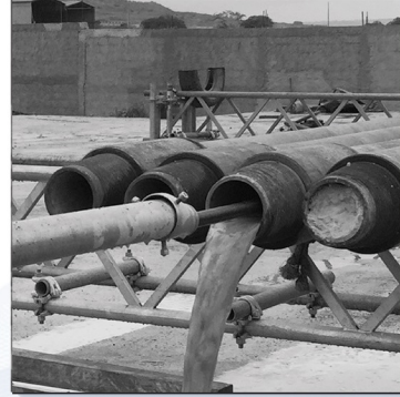
DRILL PIPE & RISER CLEANING
