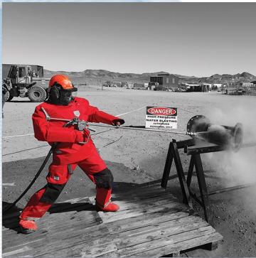
PIPE CLEANING & PIPE FLUSHING
