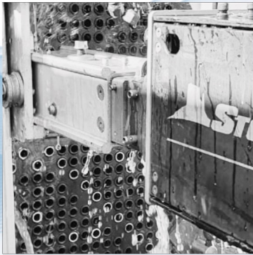
HEAT EXCHANGER TUBE CLEANING
