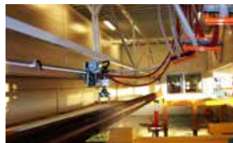
DRILL PIPE CLEANING
