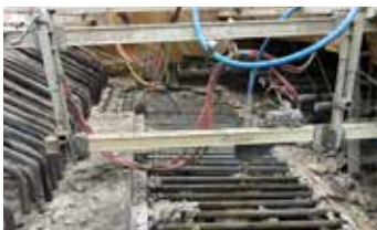
COKE AND REFRACTORY REMOVAL
